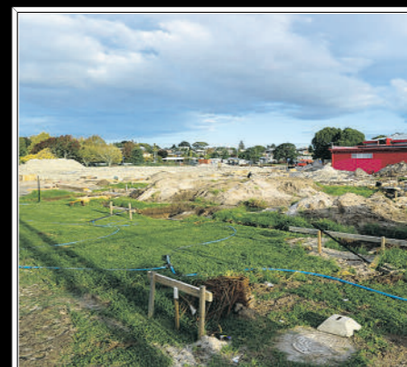
UNDER WAY: Construction has started on the new Countdown in Bureta. PHOTO/GEORGE NOVAK
